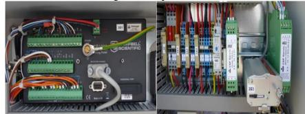
Fig. 8: Data logger. Figure 8: Connectors, GPRS modem, automatic switch [22]
